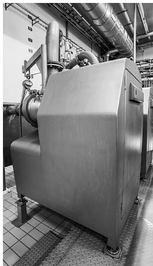
The Haarslev Pump-fed Grinder performs particularly well with softer viscous, pumpable inputs. The connected feed pump ensures a consistent flow rate that helps eliminate slippage. The consistent flow also ensures clean cutting of the material passing through the grinder, and outputs in best possible condition.
