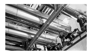
Haarslev shell & tube heat exchangers quickly and effectively bring these vapors into an easy-to-handle liquid form, using only a minimum of energy – for pumps to circulate the cooling water.
