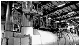
ELIMINATE ODOR PROBLEMS STEMMING FROM RENDERING AND PROCESSING MEAT AND FISH BY-PRODUCTS - AND OTHER INDUSTRIAL PROCESSES. You can quickly and effectively get rid of virtually all unpleasant odors in the gases and vapors from your rendering plant by exposing them to very high temperatures in combination with the presence of oxygen. This triggers an oxidation reaction that transforms the problematic complex organic solvents into simple, easy-to-dispose-of mixture of mainly CO2 and H20.
